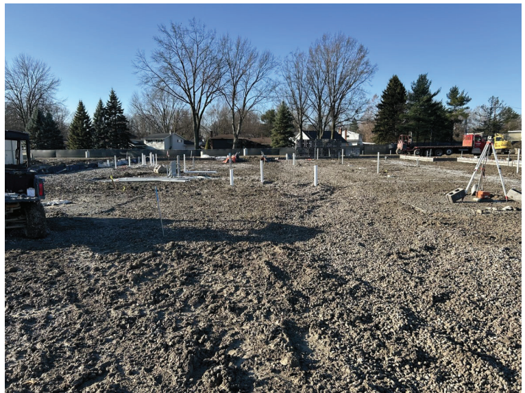
Underground Plumbing and Electrical
