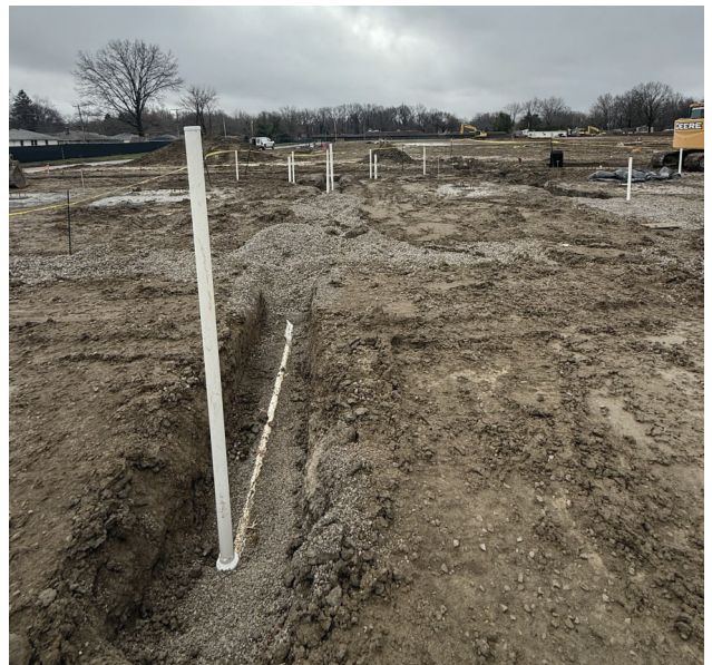
Underground Plumbing Main Corridor
